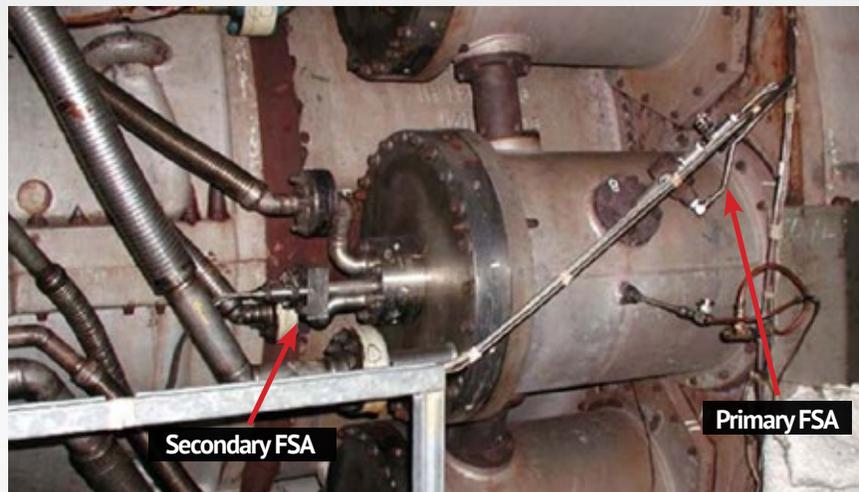
**Note:** In climates with high relative humidity or in applications where engines are operated in peaking service, a bleed air purge connection port (1/8" NPT) is included within the standard assembly and can be utilized if required. The standard assembly comes with a 1/8" allen pipe plug fitted. This feature allows compressor discharge pressure (CDP) air to be used to remove moisture from the FSA optical surfaces.
