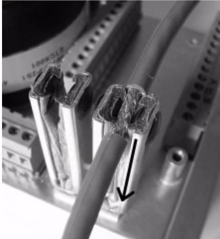
Where screened cables are required to run through one device to connect to another, terminals are provided to allow the screens to be connected, by forming a 'tail' with the braided screen of each cable, the length of unscreened cable short be kept as short as possible, but in any case **MUST NOT exceed 30mm**, per cable 'tail'.
