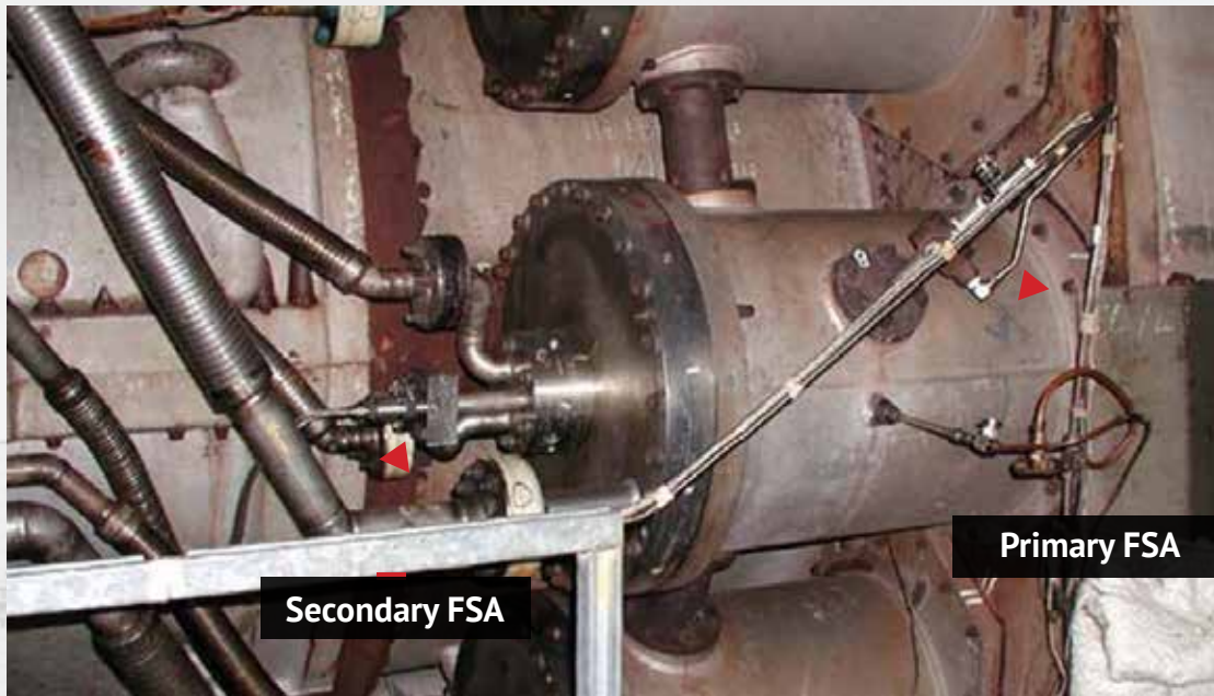
Figure 5 Frame Engine Primary and Secondary Installations
